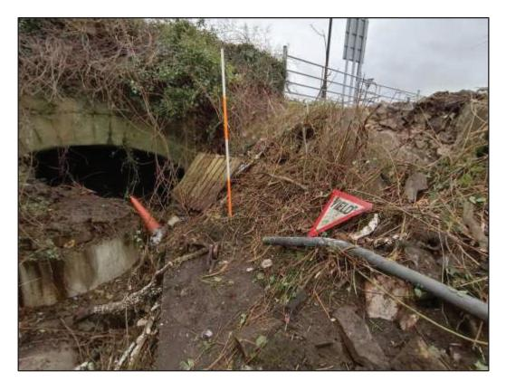
Plate 2.6: Arched culvert and watercourse with foundation level of gable of the 1865 extension to the right
